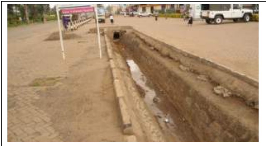
Plate 6-4: An open storm water drain in the CBD
