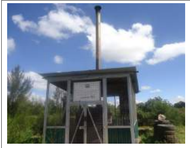
Plate 6-14: Nanyuki District Hospital Incinerator
