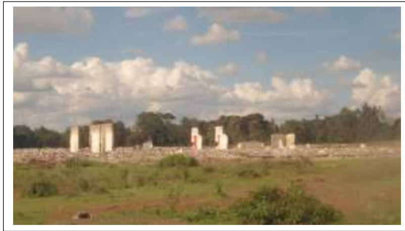
Plate 5-4: Vandalized MOUNTEX Factory
