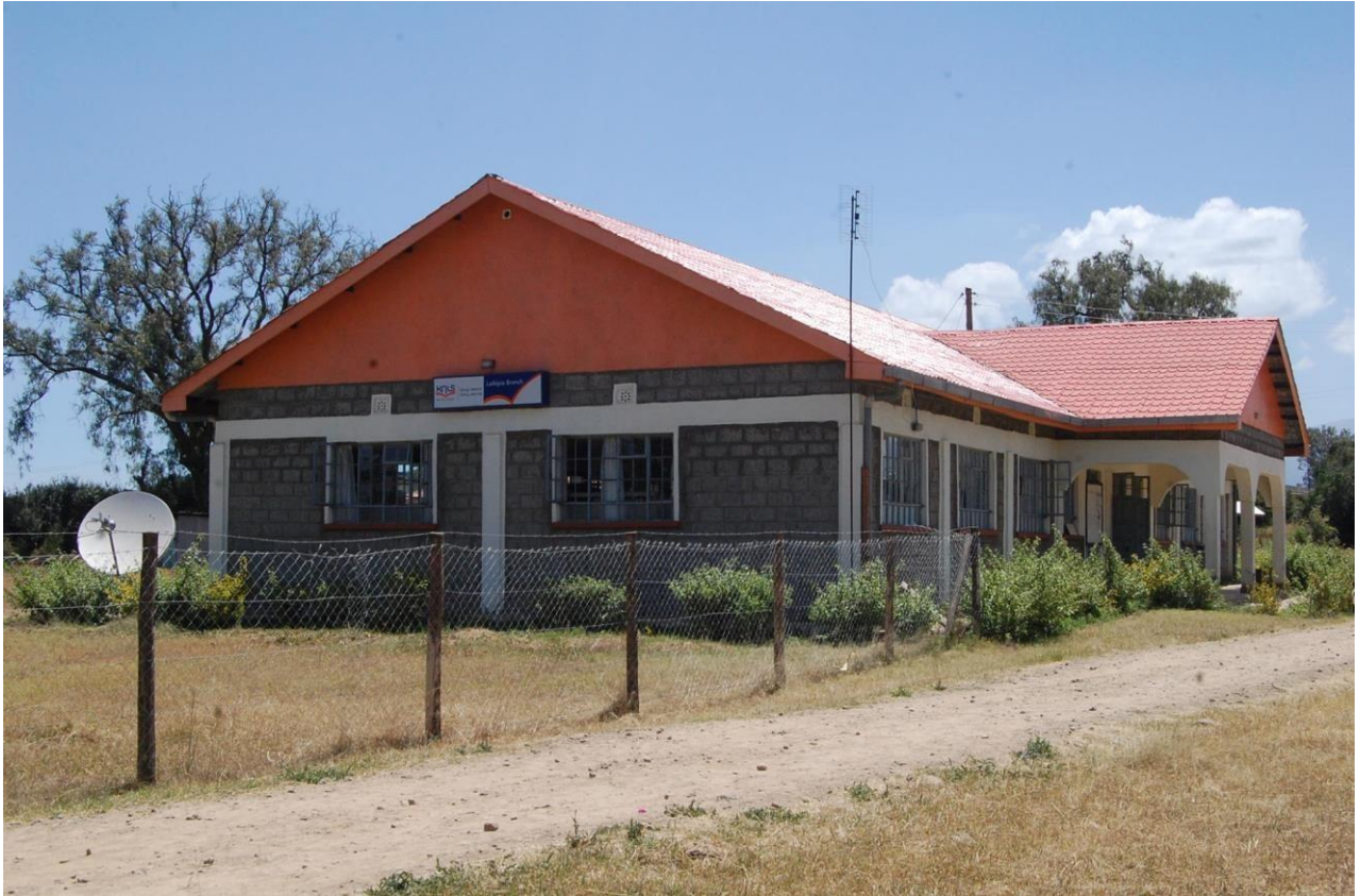
Figure 2: Existing Nanyuki Library
