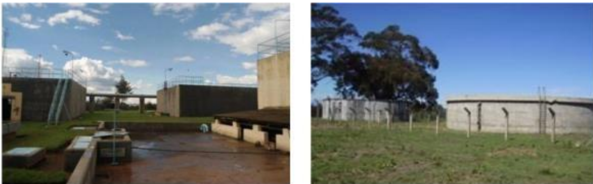
Figure 1: Water Treatment Works and Water Tanks in Nanyuki Town
