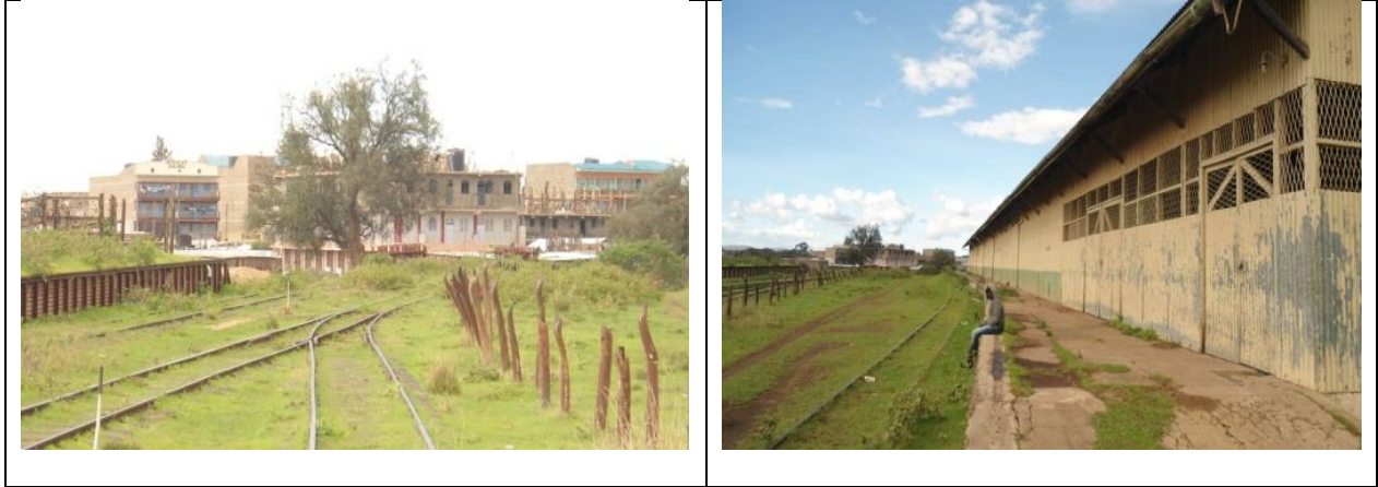
Plate 6-6: Nanyuki underutilized Railway Station
