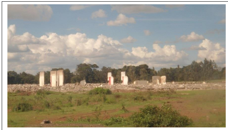
Plate 5-4: Vandalized MOUNTEX Factory
