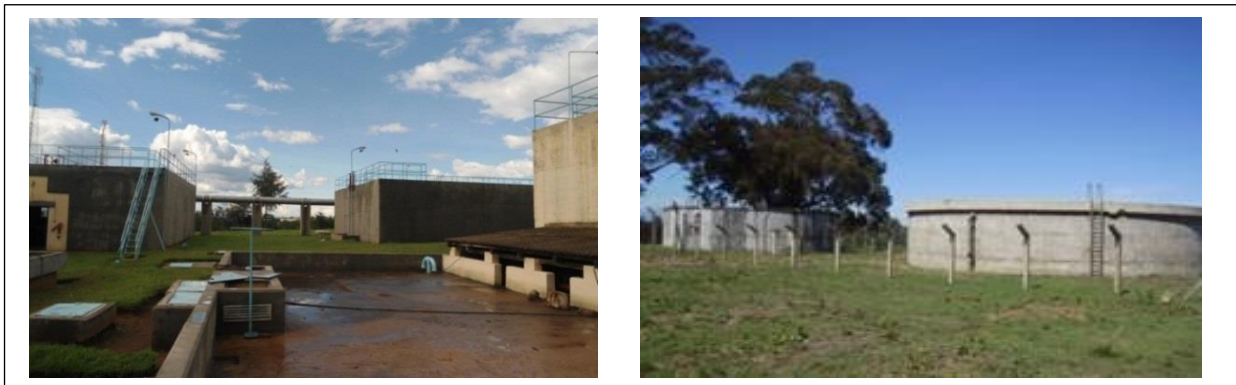
Plate 6-10: Water Treatment Works and Water Tanks in town
