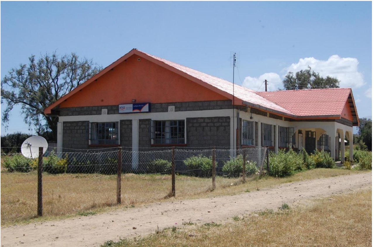
Figure 2: Existing Nanyuki Library
